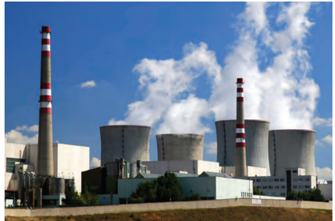
Figure 9.17 : An Atomic Power Generation Plant
