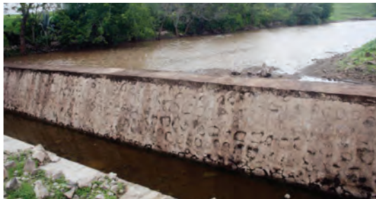
A bund on a river
