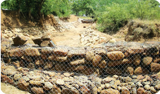
Fig. 6.12 : Gabion dam on stream
