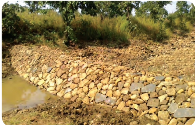
Fig. 6.11 : Loose rock check dam
