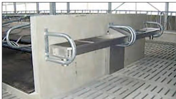
Fig. 2.18 : Modern automated water trough
