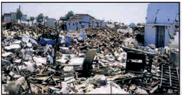
Figure 5.2 :The Bhuj earthquake 26 th January,2001
