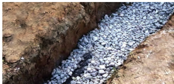
Fig 7.11 : Tile drainage
